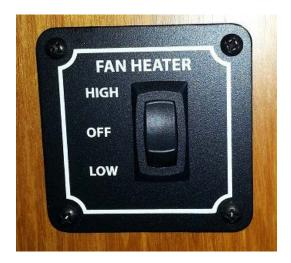
The system will run for approximately 10-15 minutes before the fans automatically start running. There are internal temperature sensors that require the coolant to be at a certain temperature before this happens.
