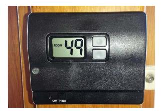
Now activate the heating system by switching the System Heat switch from the off position to system heat. The green light will be activated showing the system is on. You will hear the burner ignite which is located on the starboard of the engine room.
