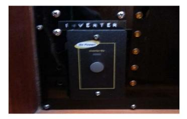
The inverter's power source is the starboard engine battery located in front of the starboard engine. The quantity of AC power is <u>limited</u> to the capacity of only this battery. Monitor your battery usage very carefully! The Five Battery Volt Meter should never indicate less than 12 volts. When the inverter is not being used for heat or TV/DVD turn it off.
