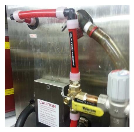
Make sure the water diverter valve is in the direction shown. This allows water to go directly from the Everhot tank to all hot water faucets throughout the boat. When docked and utilizing electric power and the electric hot water tank, return the directional valve to the electric engine position.
