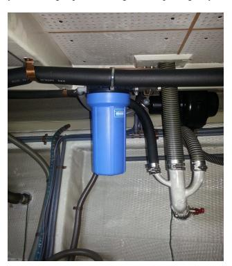
Water will escape and drain down through the bilge. Replace the filter with the new one and reattach the filter housing securely to prevent any leaks.
