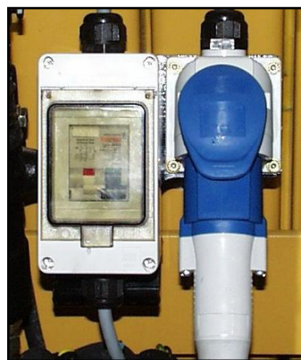
Fig. 8.2 - 220V electrical power socket and circuit breaker.
