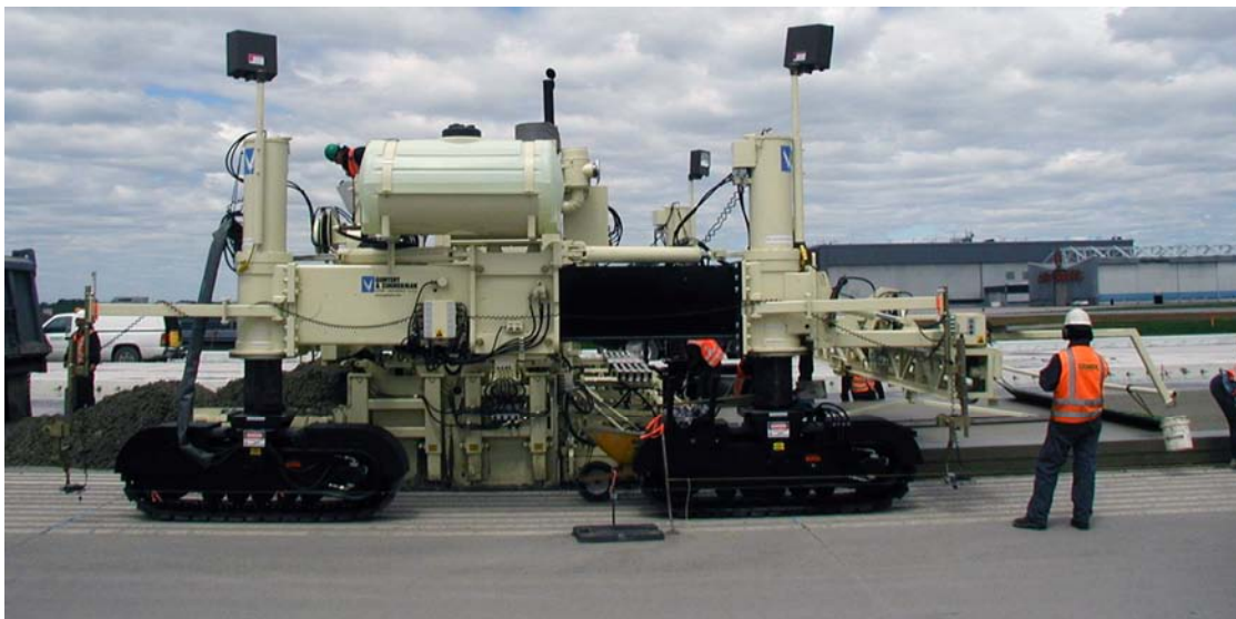
Figure 22. Side forms should be parallel to the stringline.
