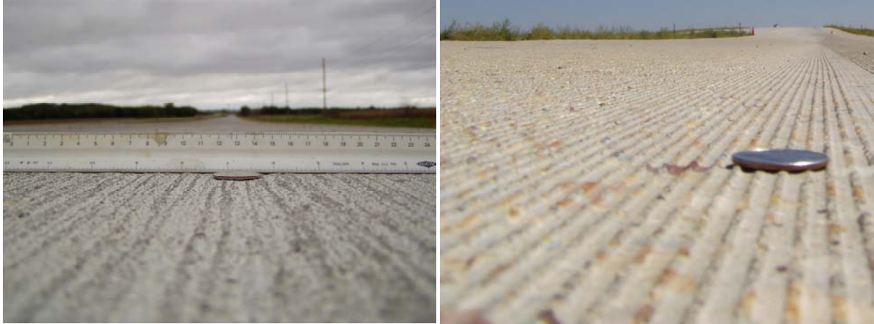
Figure 5. Drag textured and diamond ground concrete pavements.
