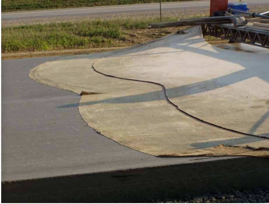
Figure 39. Burlap drag attached to a work bridge.
