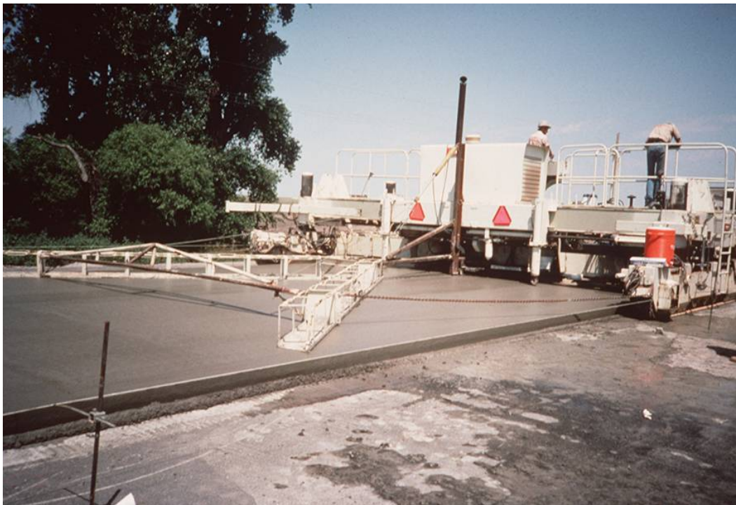
Figure 29. An alternative chevron-type float attachment for a paver.
