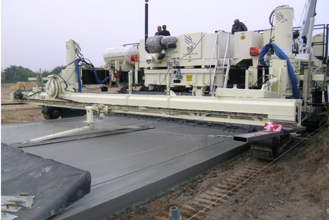
Figure 28. Automatic longitudinal float attached to the back of a paver.
