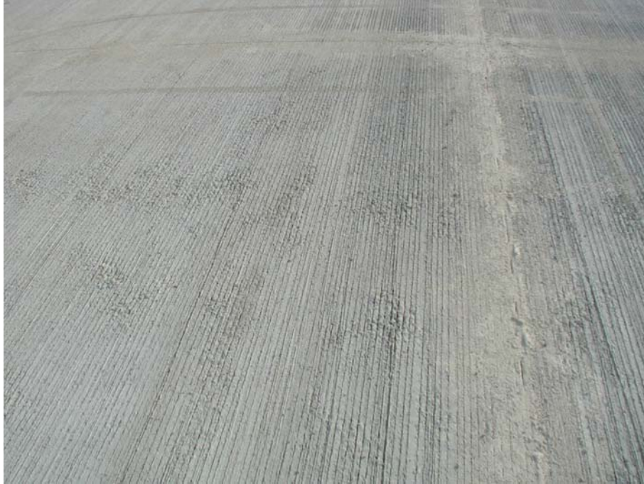
Figure 13. Variability in tined texture due to mix segregation/consistency problems.
