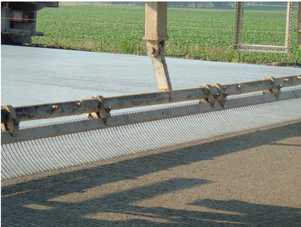
Figure 6. Longitudinal tining of a newly placed concrete surface.
