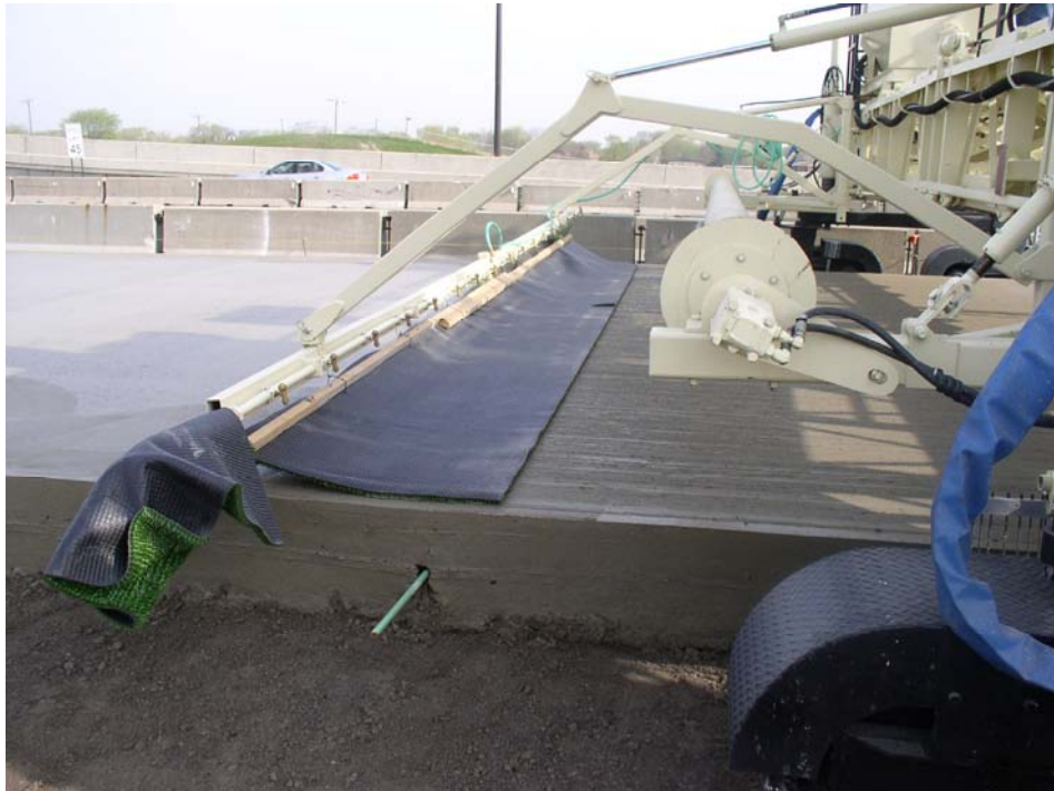
Figure 38. Turf drag attachment on a texture machine.
