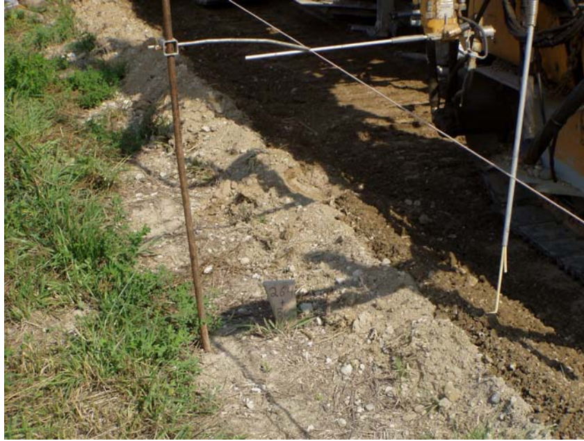
Figure 21. Sensor rods that track alignment and elevation.
