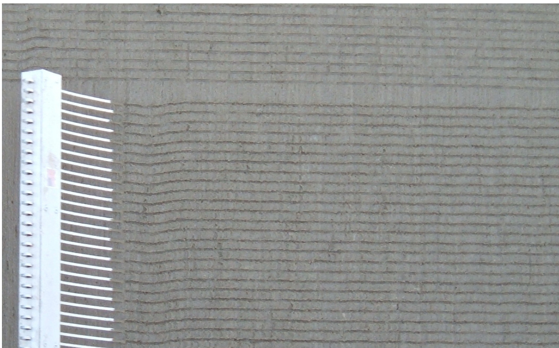
Figure 17. Transverse start/stop point matching.
