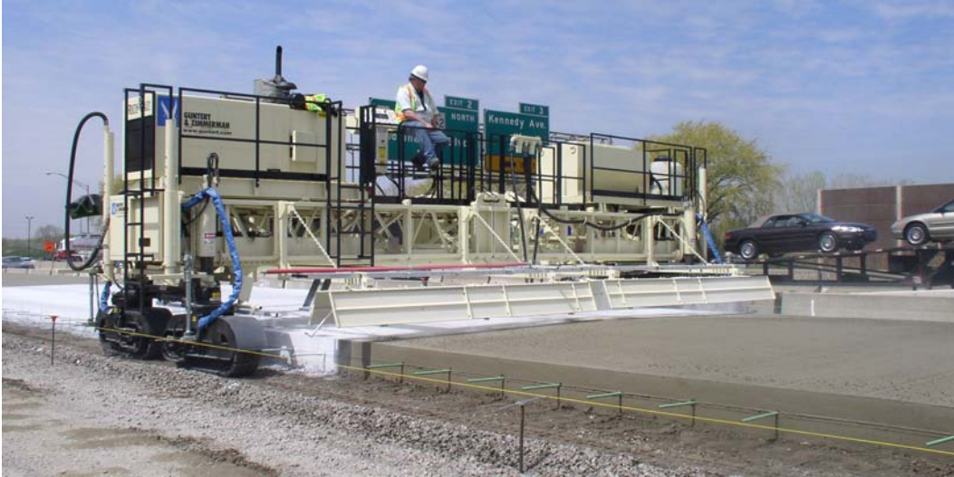
Figure 32. Texture-cure machine manufactured by Guntert & Zimmerman.
