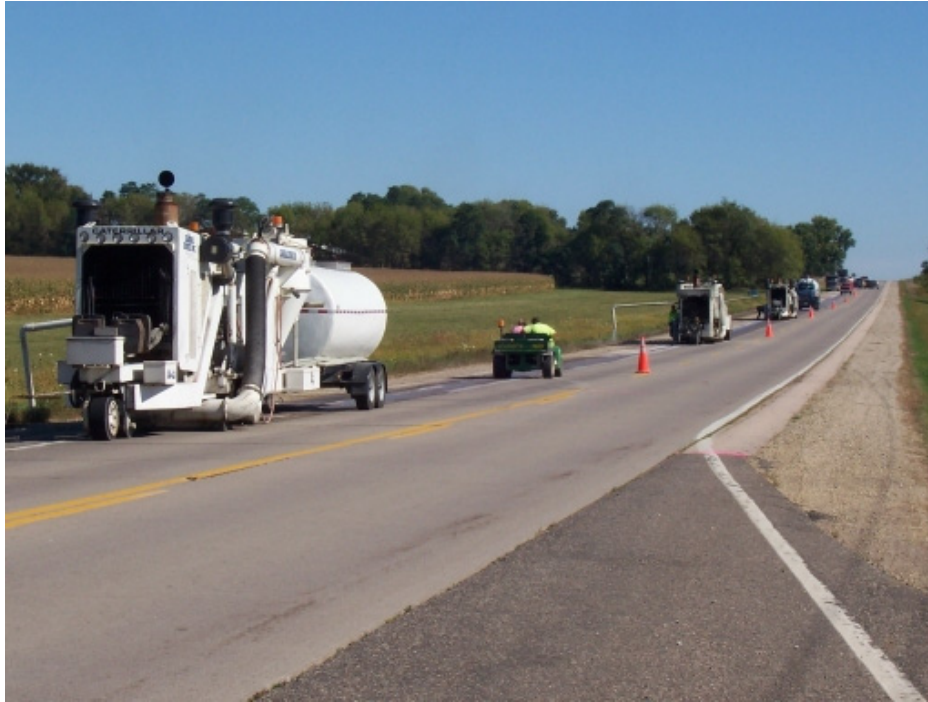
Figure 1. A grinding large-scale concrete pavement resurfacing operation.
