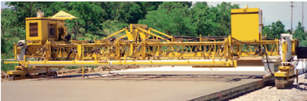
Figure 33. Texture-cure machine manufactured by GOMACO.
