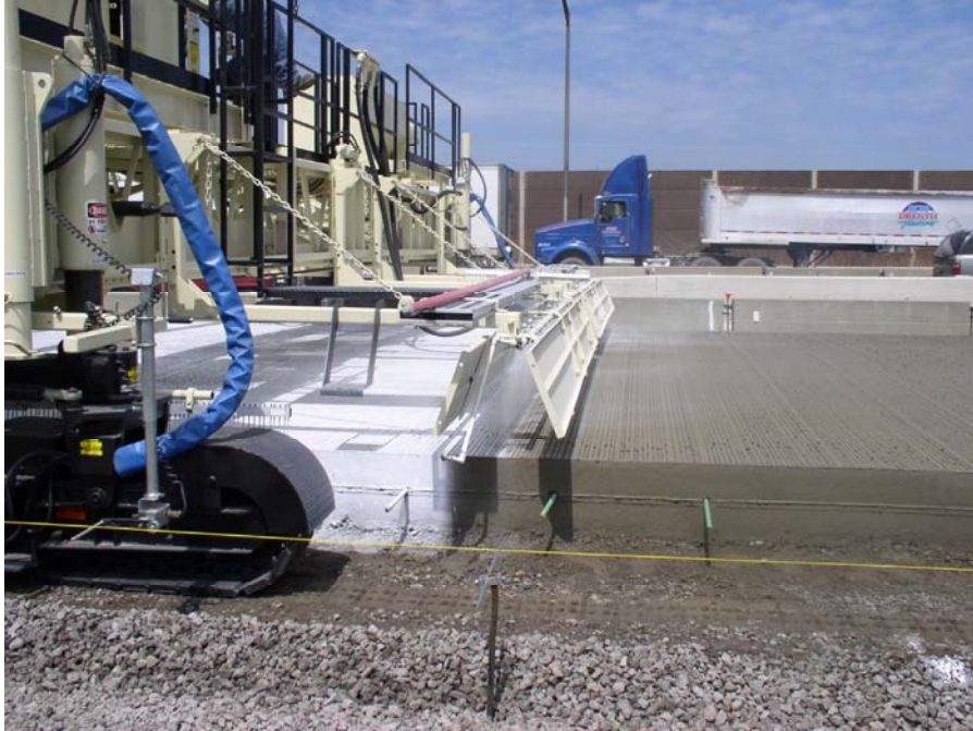
Figure 42. Illustration of curing equipment on texture-cure machine.
