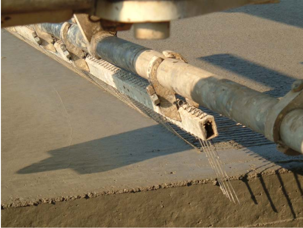
Figure 14. Angle of tines affecting contact with concrete surface.
