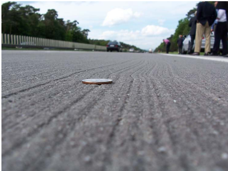
Figure 15. Deep striations from burlap drag used on an Autobahn highway in Germany.
