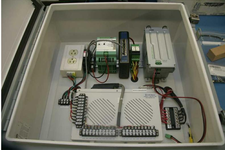
*Insert the three power wires into the A/C power input, located on the middle left-hand side of the unit*
