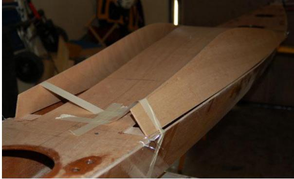
Masking tape holding the deck side panels in place while wiring.
