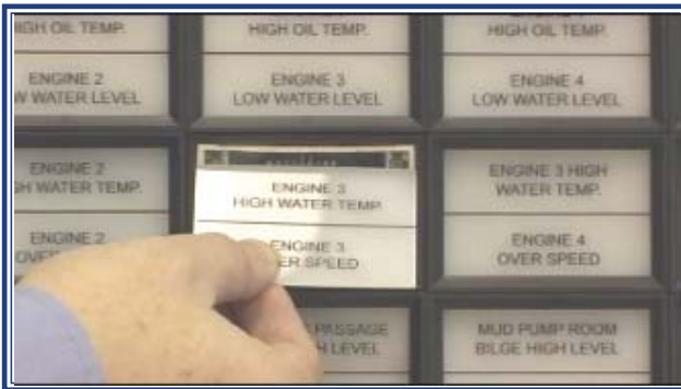
6- Place the new lens inside the frame
