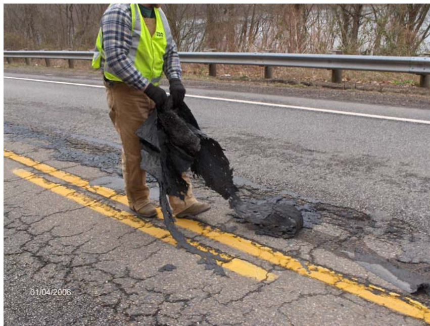
Figure 4-4 Example of liquid asphalt applied to a damp road
