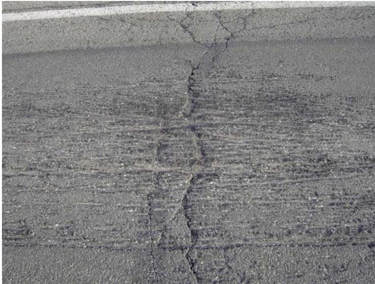
Figure 1-9 thermal cracking
