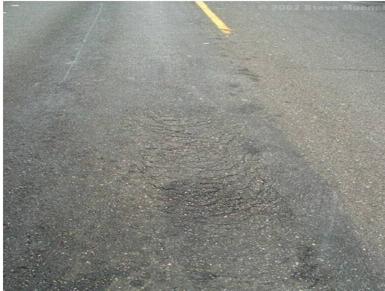
Figure 1-8 slippage cracking
