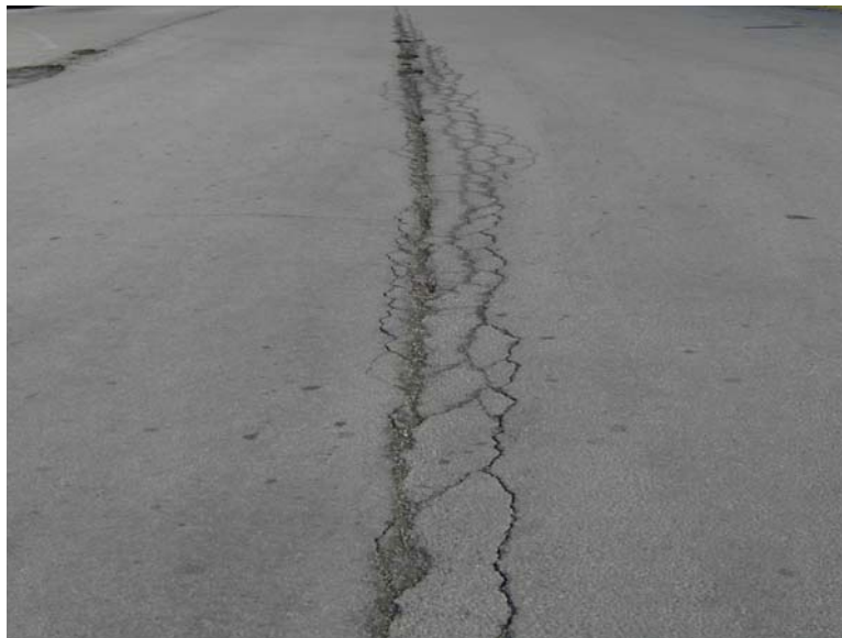
Figure 1-7 joint cracking
