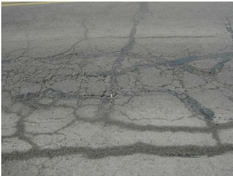
Figure 1-10 alligator cracking
