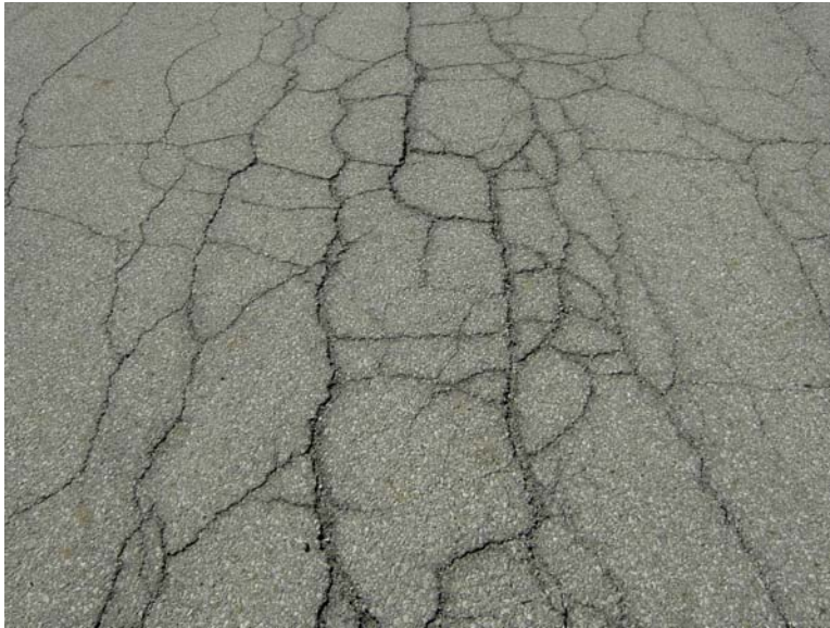
Figure1-5 block cracking
