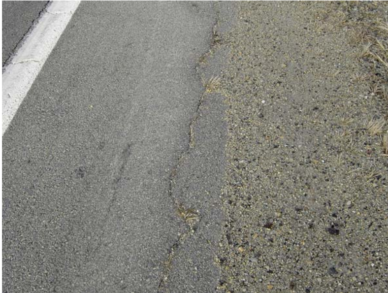
Figure 1-11 edge cracking
