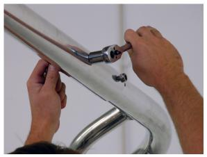
Once all the holes are drilled and all the fasteners are inserted the nuts can be installed and all of the fasteners and nuts can be firmly tightened.
