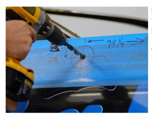
If necessary, you should move the wires out of the way while you drill. We recommend drilling a small pilot hole which will keep the 5/8" drill bit from walking (moving). A small rat tail file can be used to ease the edge and keep the gel coat from chipping. Be careful of wires!
