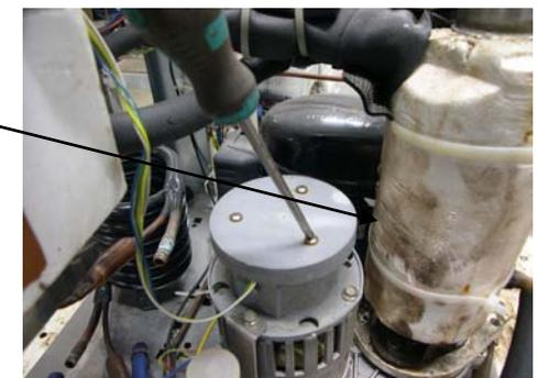
2. REMOVE THE PLASTIC STORAGE OF THE MOVEMENT SENSOR.
