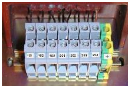
Details of current transformers casted terminal boxes
