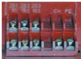
Details of current transformers casted terminal boxes
