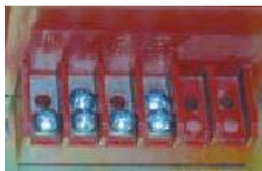
Details of current transformers casted terminal boxes
