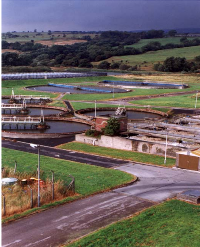
Sludge Blanket Monitoring System
