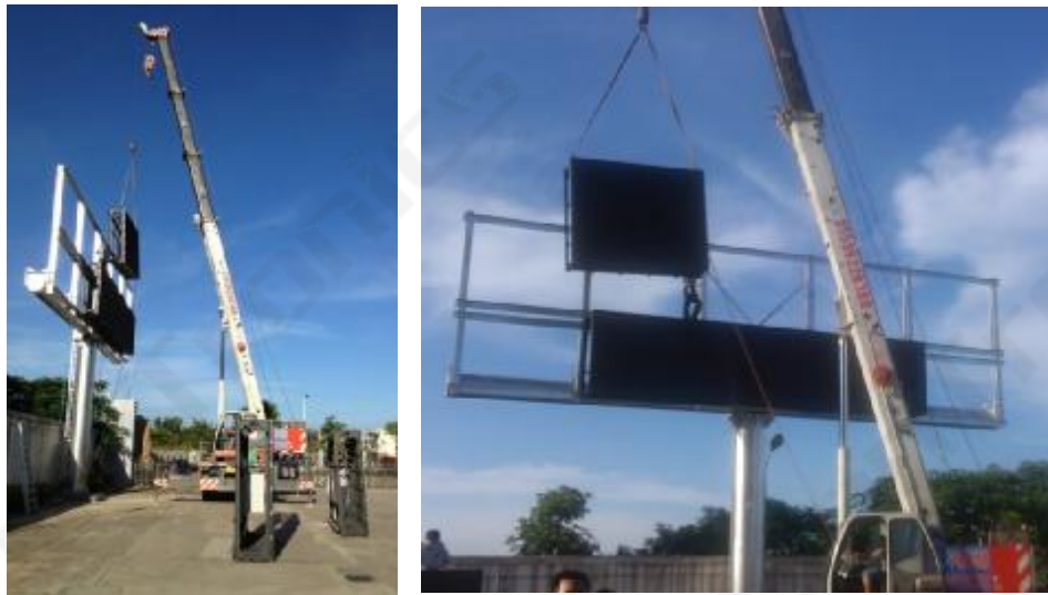
Image 4-6 The installation process of T series LED display
