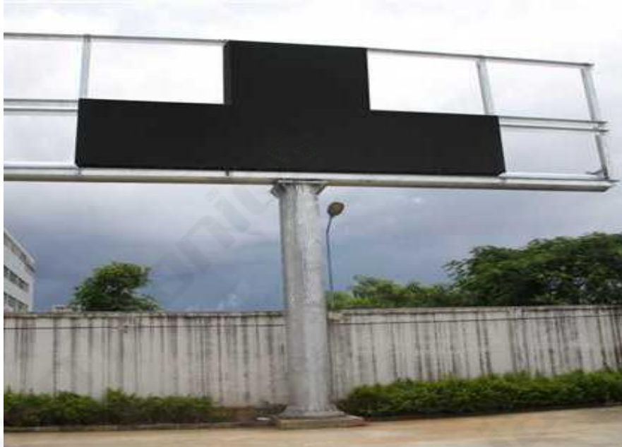
Image 4-4 Assemble the tiles from left to right and bottom to up
