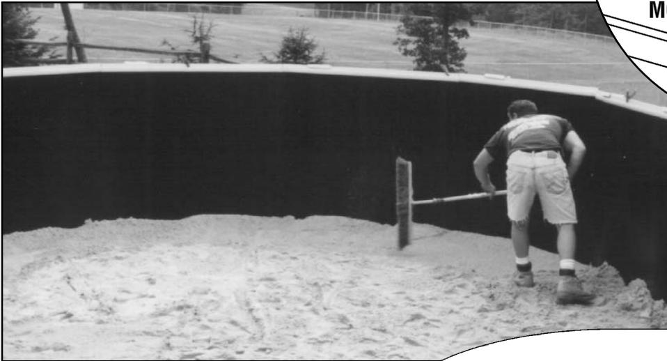
Build earth mound on top of wall guard using screened damp earth or pre-washed sand.
