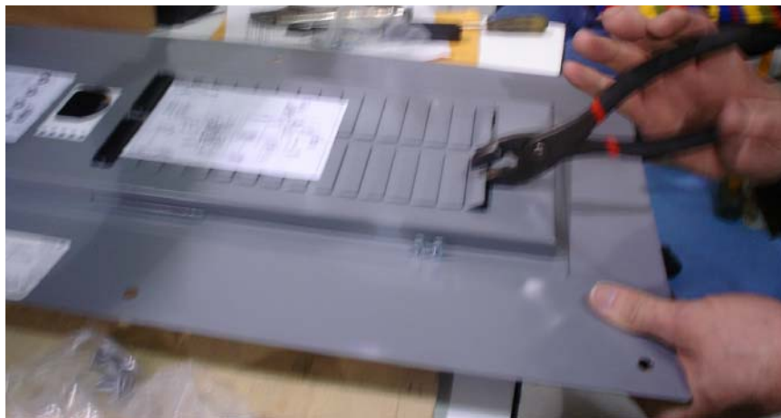
Pliers used to remove knockout from back of door mechanism
