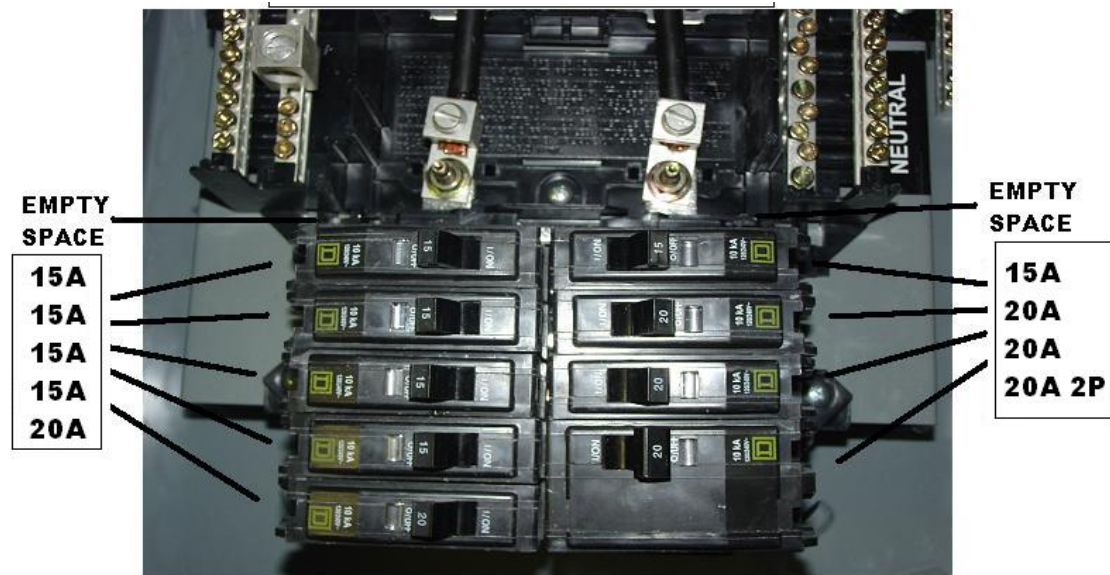
FIGURE 2: Standard Circuit Breaker Ratings/Locations
