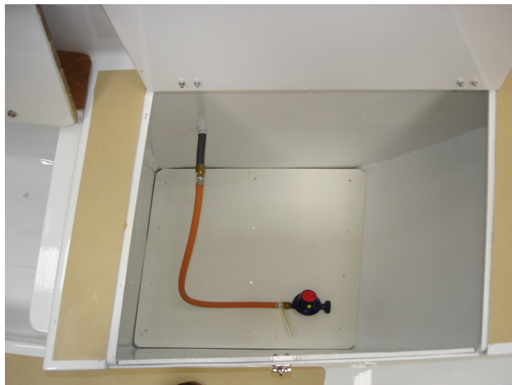
Gas Deck in starboard bathing platform
