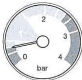
(Fig 2) requires re-pressurising
