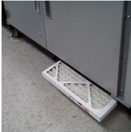
Figure 5-17 Purolator Hi-40 System Filters
