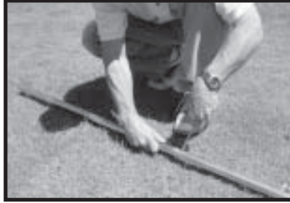
2- Insert small screw and lock washer and tighten. Repeat this procedure with all poles.
