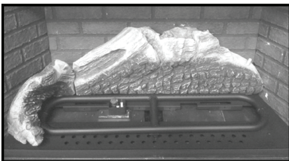
Figure 73: Rear logs 1 and 2 installation.
