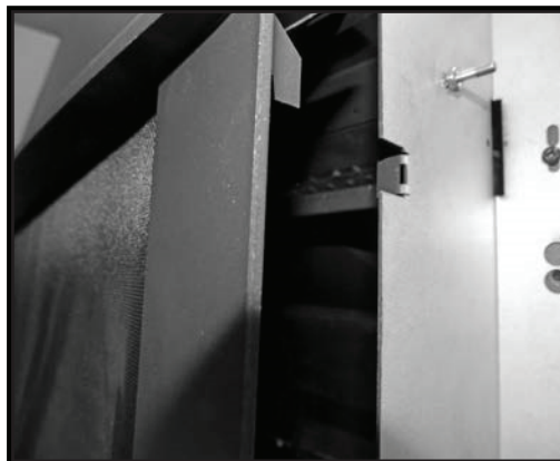
Figure 35: Surround and lintel tab.
