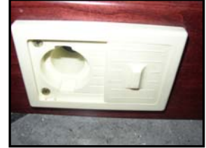
Figure 14-10. Vacuum Hose Coupling
