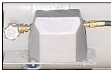
Figure 2-6. LP Gas Regulator
