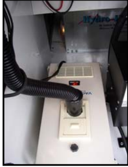
Figure 14-11. Vacuum Cleaner System
