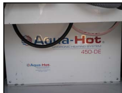
Figure 4-13. Hydraunic Heating System
