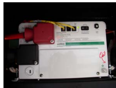
Figure 7-14. Inverter/Converter
