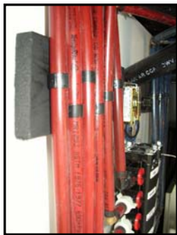
Figure 11-9. Plumbing Manifold
