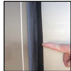
Figure 14-6. Inspecting Slide Out Gasket
