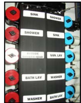
Figure 11-10. Plumbing Manifold
