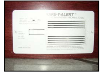
Figure 3-8. CO/LP Gas Detector
