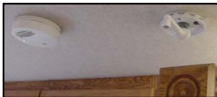
Figure 2-8. Smoke Detector (Left)
