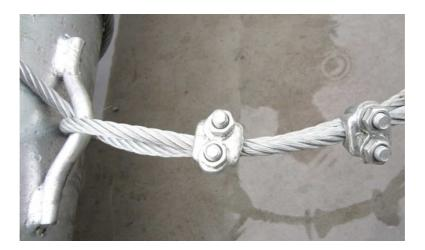
3. Besides aiming the steel wire for front basement, the ends of all other steel wire need to connect with the corresponding basement. And you could fix all wires after the installation of the tower as below:
