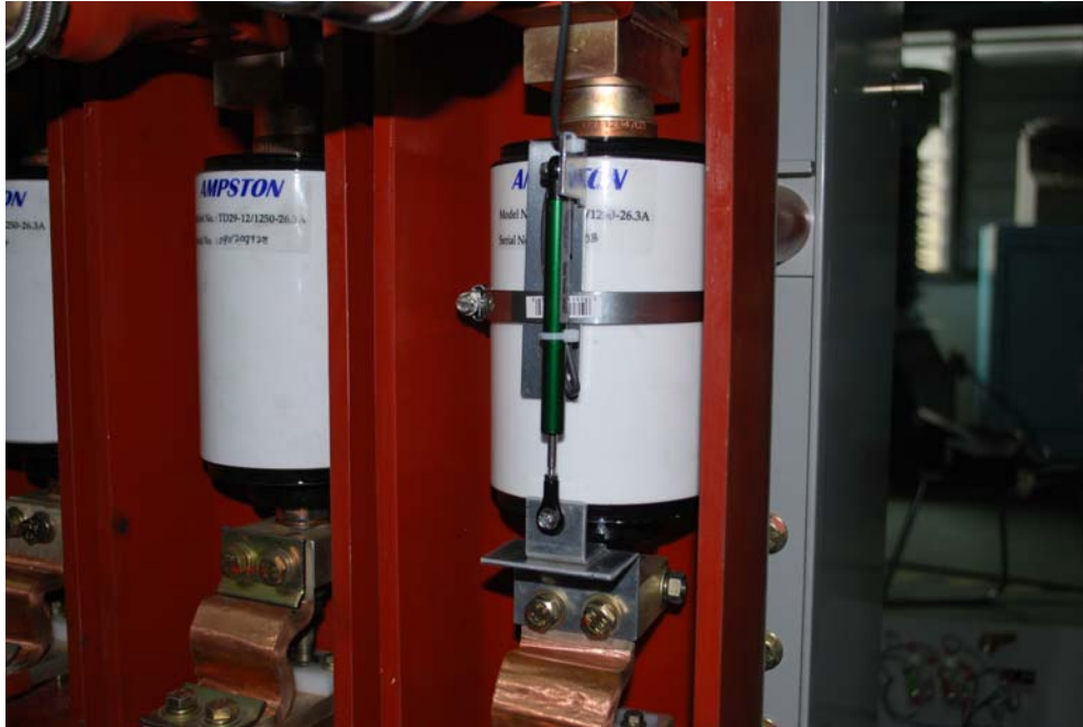
Resistor Transducer on Vacuum Circuit Breaker
