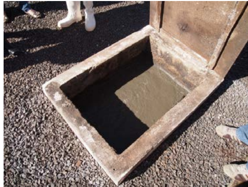
Image 31: Outlet after the main fermenter
