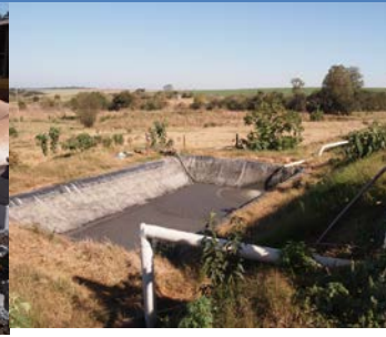
Image 28: Storage tank (secondary storage tank)
