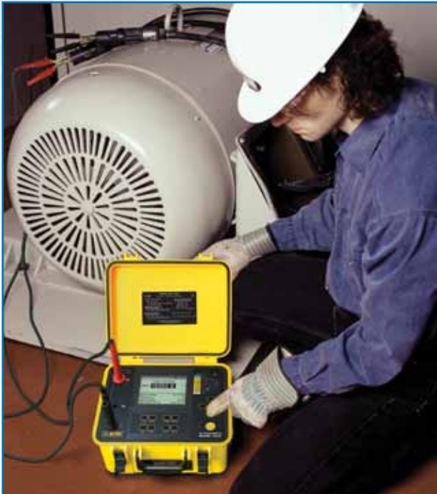
Model 6555 checking insulation resistance on feed cables to a three-phase motor.
