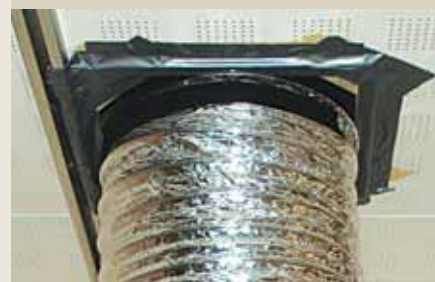
FIGURE 10 A return grille adapter with flex duct attached.
