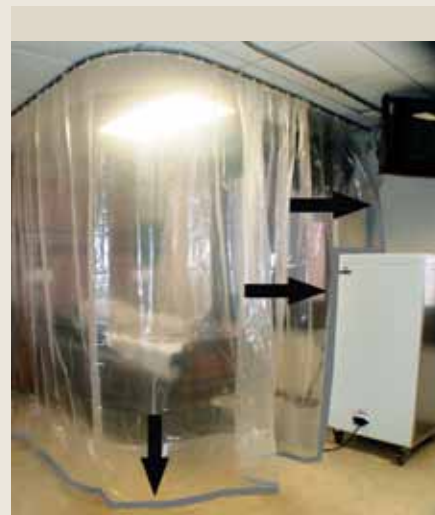
FIGURE 17 Plastic curtain taped to wall.
