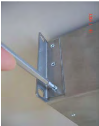
Figure 1: Rack angles assembly
