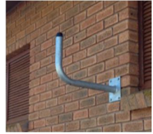
GPS antenna mounting bracket
