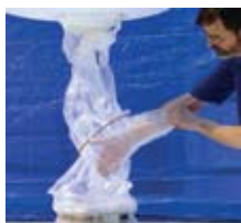
Attach liner then bag out stub
