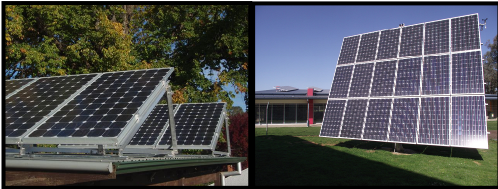
Frames used on a flat roof to correct tilt and orientation.
