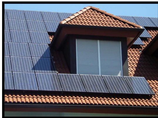
Shading of panels from the projecting roof line will affect the system's generation capacity.
