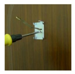
Step 3. Put the screw go through the hole on metal bracket, and screw up it to the inner screw hole on the outdoor part barrel, until fasten the outdoor part to the metal bracket
