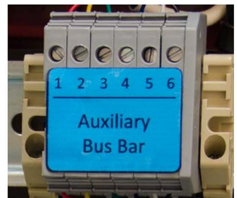
Fig. 9 - Auxiliary Bus Bar
