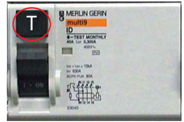
A differential-current switch with an indicated test button
