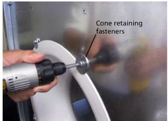
Figure 30: Fan wheel/cone alignment – Step 8
