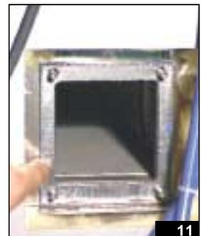
Check that the burner flange sealing gasket is in good condition and replace if worn (fig. 11).
