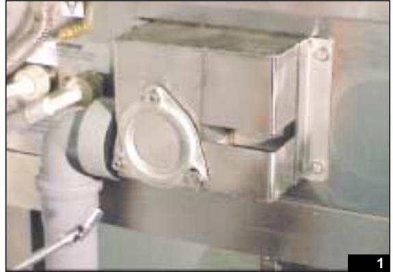
For the M versions it is imperative to fit a drain cup so as to ensure a minimum air drop of 25 mm between the plastic drainage bend of the appliance and the drainage piping. **Direct connection is not permitted.**
