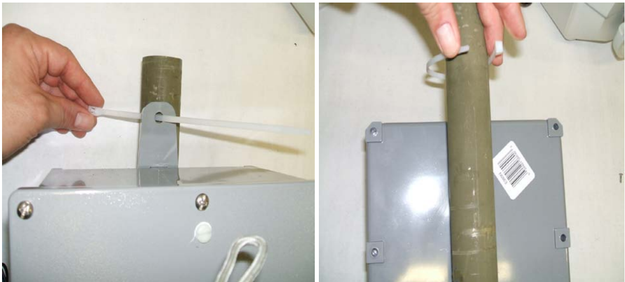
Figure 15: Using Wire Ties to Mount the Remote Transmitter Module
