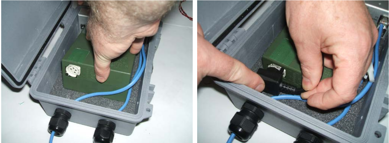
Figure 11: Installing the Military Battery
