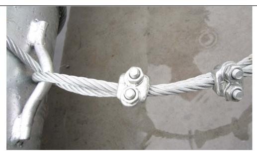
3. Besides aiming the steel wire for front basement, the ends of all other steel wire need to connect with the corresponding basement. And you could fix all wires after the installation of the tower as below
