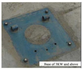
Put the edge anchor into the edge basement, and check the distance between the hook and the center as well as the basic level, and then pour the concrete. Picture is as below.
