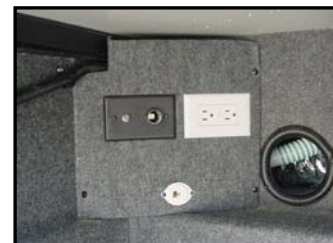
Figure 4-17. Cable & Telephone Jack
