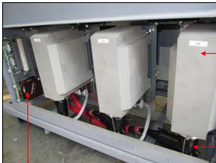
Choke coil and resistor (anti ferro resonance filter)
