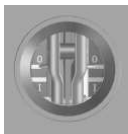
Figure 4-7: Change-over switch in the earthed position
