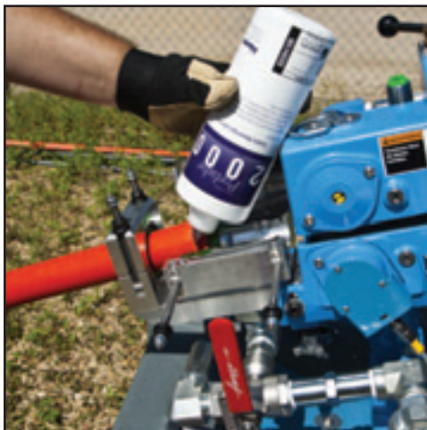
Figure 52. Add Lubricant before Cable Assembly
