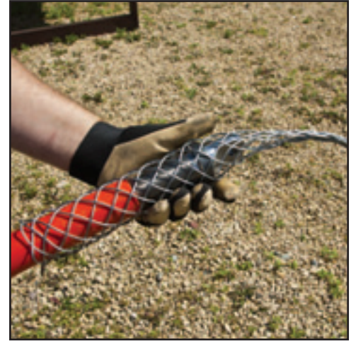
Figure 29. Installing Pulling Grip
