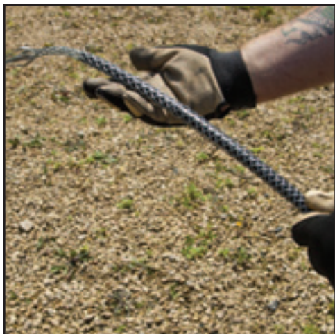
Figure 46. Install Cable Grip on Fiber Optic Cable
