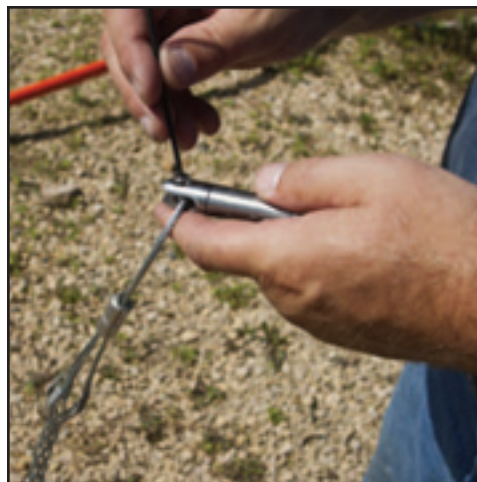
Figure 47. Install Swivel on Cable Grip
