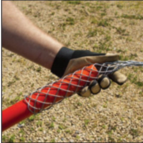
Figure 35. Install Pulling Grip on Conduit
