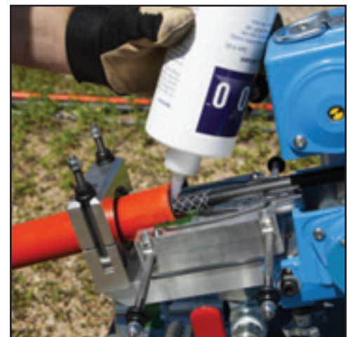
Figure 54. Add Lubricant Behind Cable Assembly
