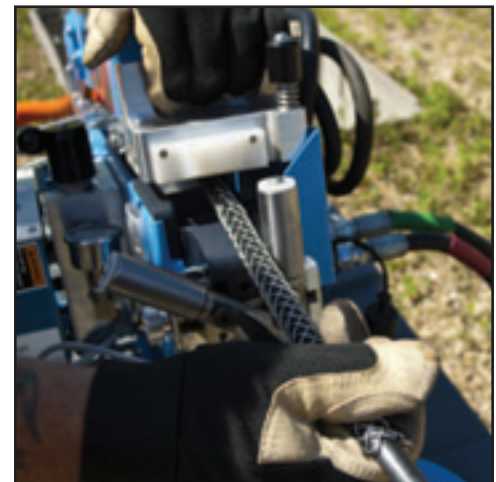
Figure 53. Feed Cable Assembly Through Blower
