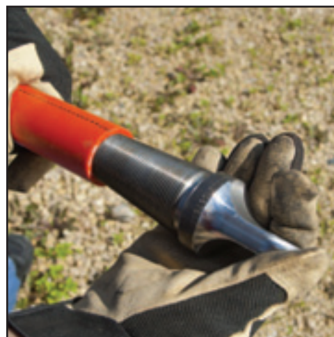
Figure 7. Installing Conduit Pulling Eye
