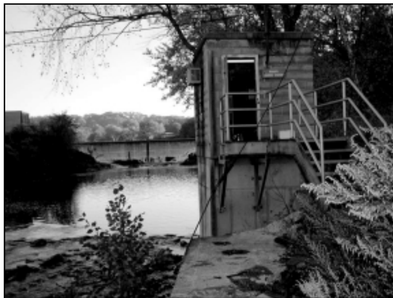
Figure 1. Flow-through water-quality monitoring station. (PHOTOGRAPH: RAMAPO RIVER AT POMPTON LAKES, NEW JERSEY, BY MICHAEL J. DELUCA)
