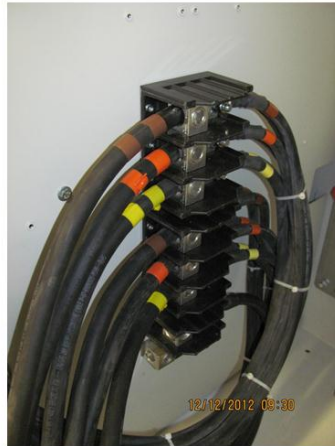
Figure 3-6: Isolation Transformer Wiring BIGI-250
