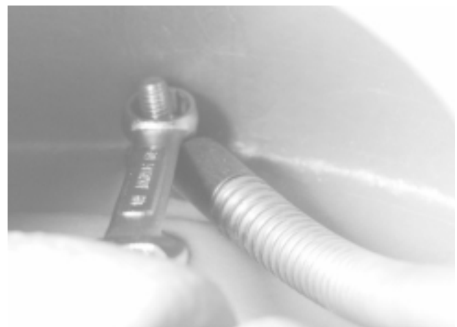
Figure 14 – Removing Pigtail Anchoring Bolt
