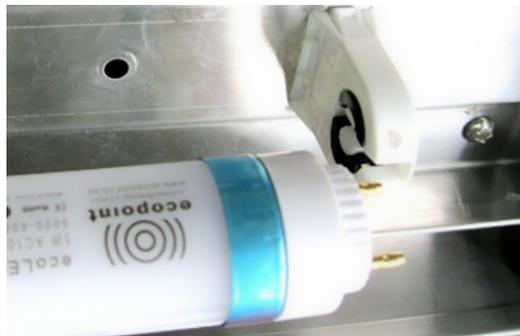
4. Fit a new LED tube and clip the diffuser back into place. Reconnect to the power supply.
