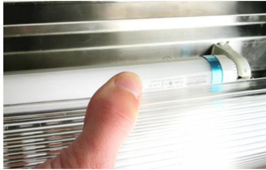
3. Rotate the LED tube until the pins on the ends of the tube align with the slots, then slide it out.
