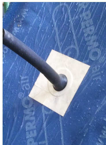
Figure 7: Sealing of the Roof Underlay using the self adhesive sealing collar .
