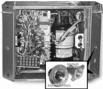
Figure 12: Water connections - small ton
