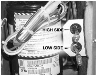
Figure 11: Schrader connections
