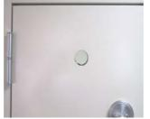
**Step2:** If no hole created from door yet, please drill the hole from the door (Recommend 165  $\sim$  175 (CM) height depends on practical application) which diameter size range of hole size estimated recommend are between  $\psi$  3.5 $\sim$   $\psi$  4.2 (CM)
