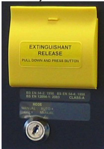
One or two key-switches can be fitted to the panel.
