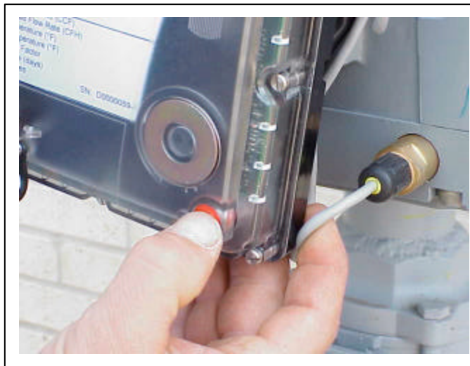
Figure 7.14 Security Seal Replacement
