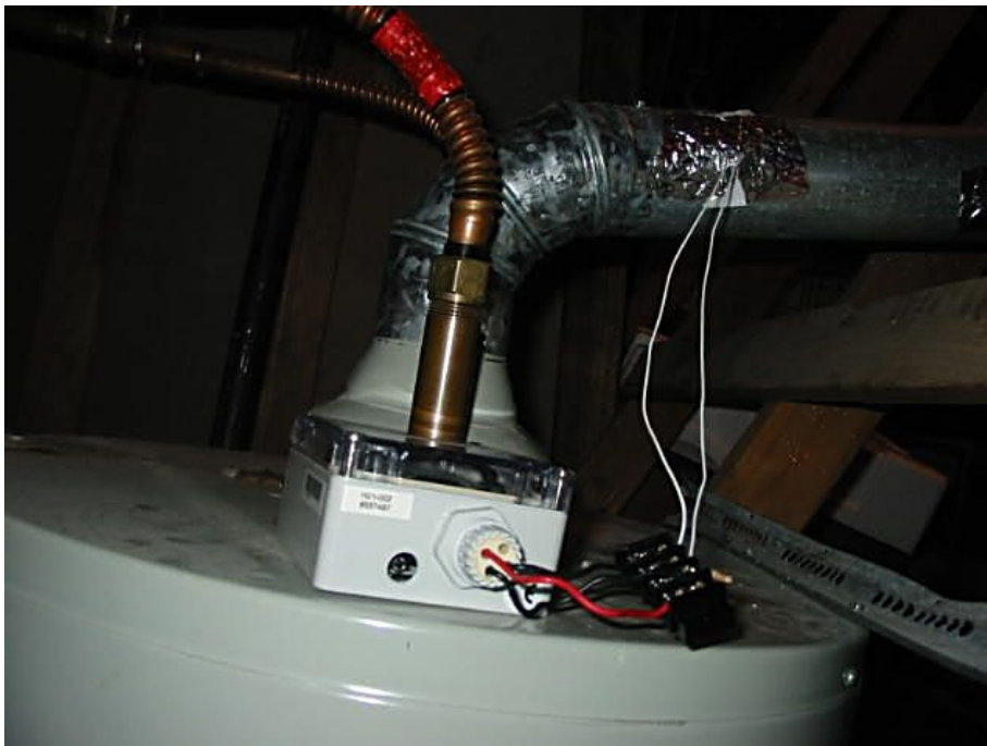
Figure B-18: Domestic Hot Water Data Logger Installation
