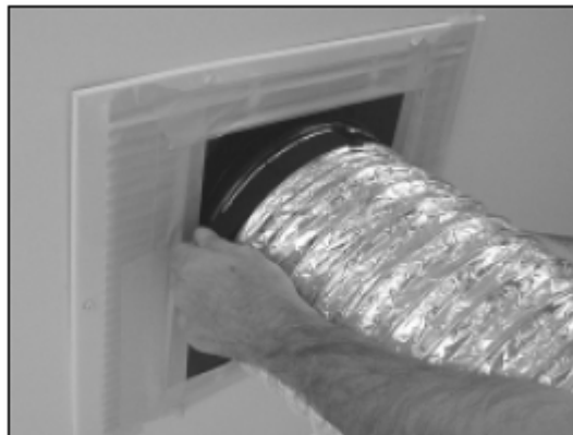
Figure B-9: Installing the Duct Blaster
