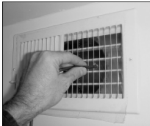
Figure B-11: Placing Static Pressure Probe in Supply Register
