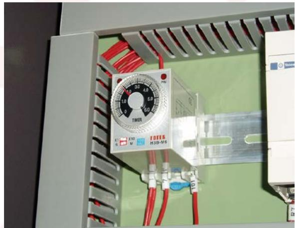
(This timer controls the oil supply interval. The factory setting of oil supply interval is once per 3 minutes. If the amount of oil is to be increased, the interval shall be shortened)
